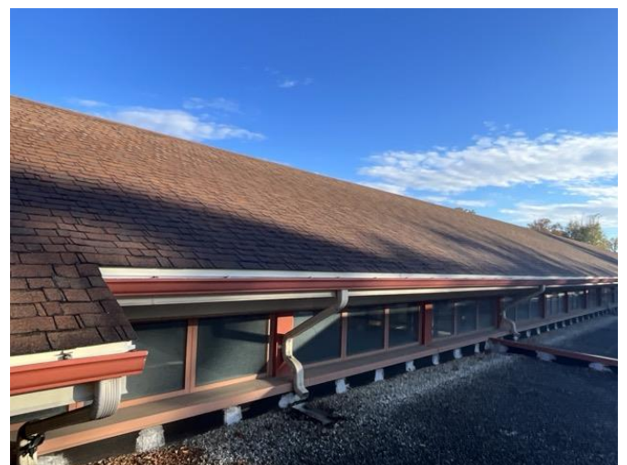
6 - ASPHALT SHINGLE ROOFING
