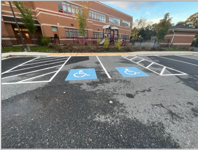
OVERVIEW OF ACCESSIBLE PARKING AREA
