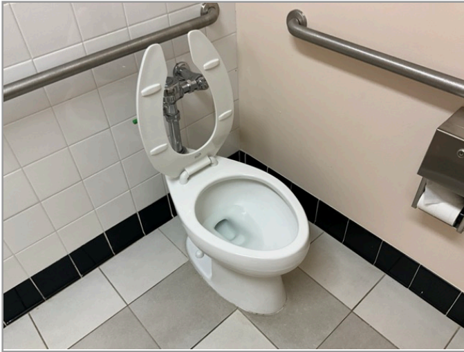
TOILET STALL OVERVIEW
