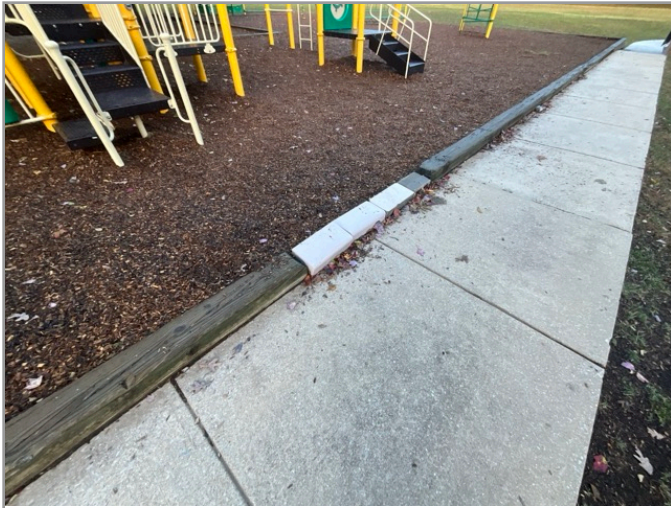
ACCESSIBLE ROUTE TO PLAYGROUND
